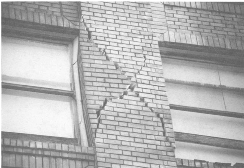
Figure 9. Cutting damage on the wall edge of the gaps [20].
