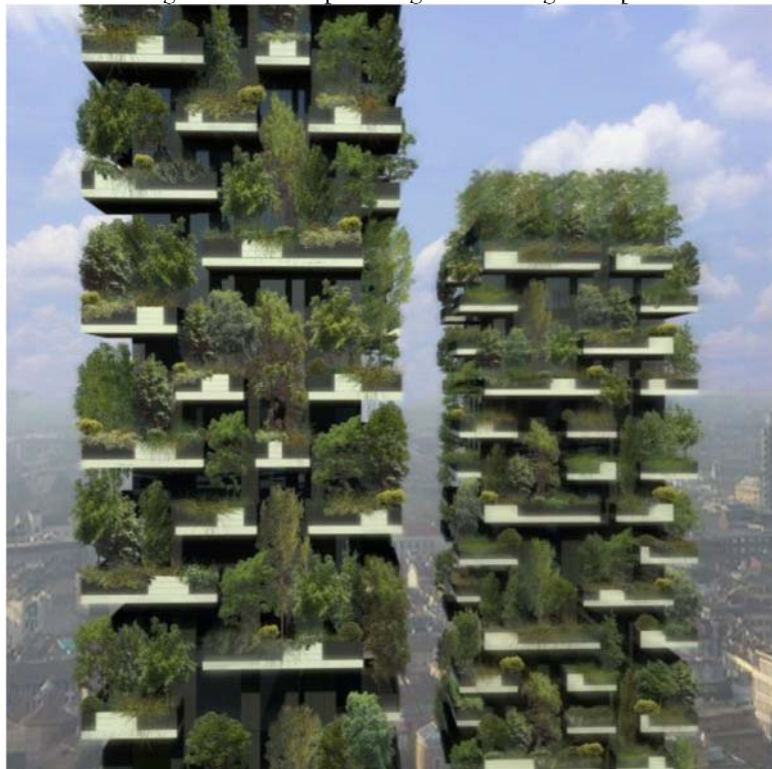
Figure 3. Vertical forests in Milan, Italy – banking on “eco” as the new fashion
