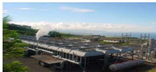
• Figure 9. Two-phase binary geothermal power plant.
